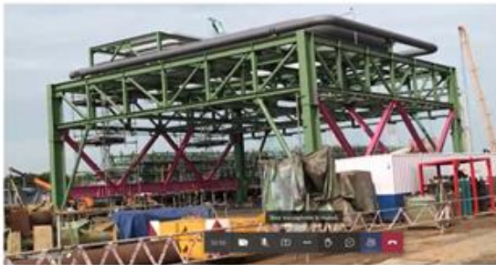
Steel structure in India's fabrication yard
